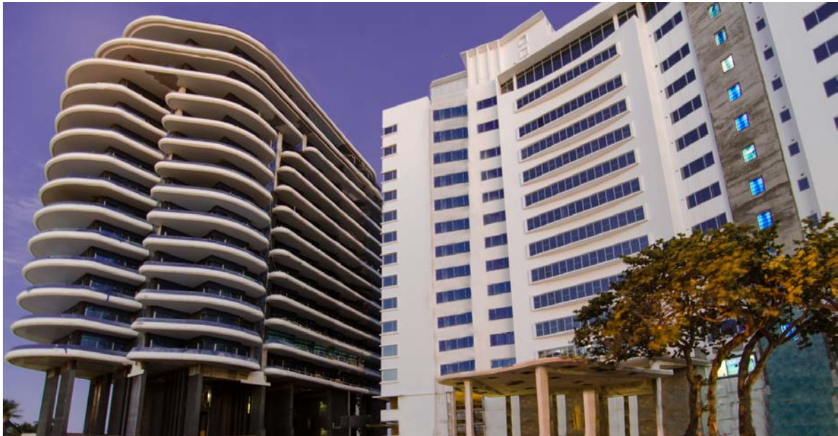
FAENA HOUSE SAXONY HOTEL (RENOVATION)
