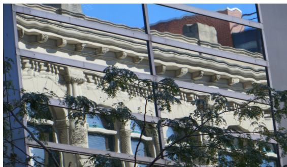
Illustration 51: Roll Wave Distortion in Architectural Glass installed in a Building
